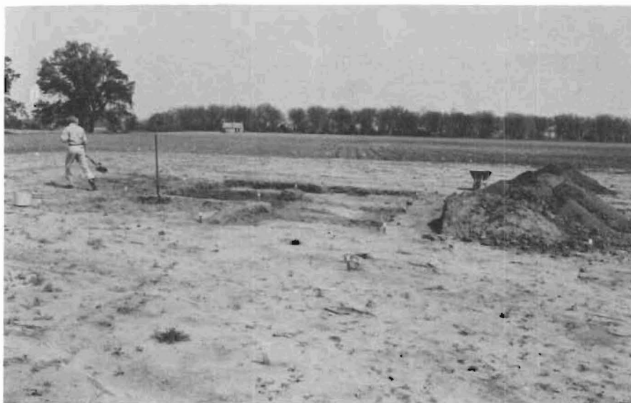
Plate 28. Clover Hill Site: excavation of House 1.
