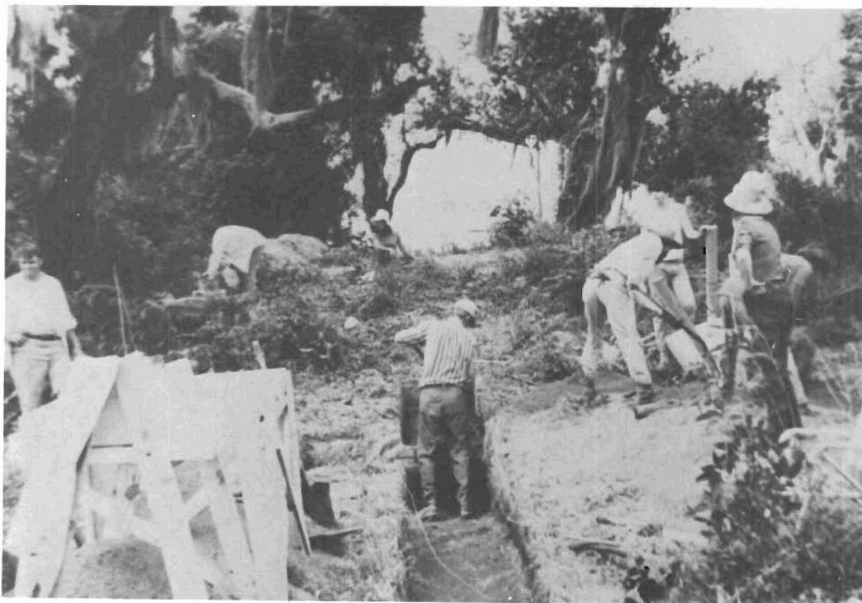
Plate 10. Jackson Landing-Mulatto Bayou Earthwork: view of excavation.
