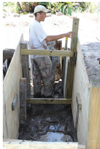
Figure 4-32. Building the cofferdam in N169E8.
