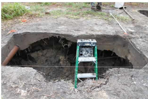
Figure 4-11. Collapsed walls of unit N171E6, facing east.
