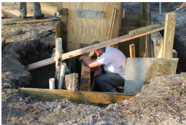
Figure 4-35. Upper portion of the shoring and bracing in N171E6.
