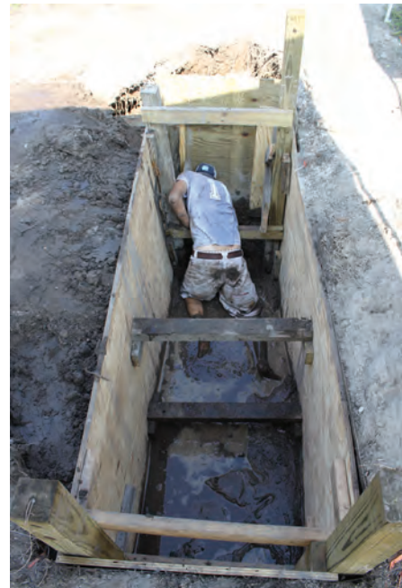
Figure 4-15. Excavations in N168E6 after Hurricane Alex.
