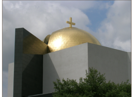
Figure 3.3C. Gilded copper dome crowns the Chapel of St. Basil in Houston, Texas; Niko Contracting, sheet metal installer.
